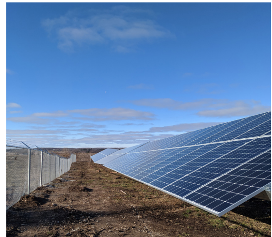
Project MS05, a 600kW DC project completed in December 2020.
